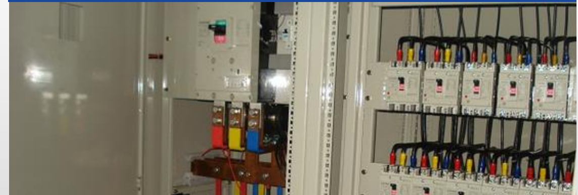
Power supply installation according to design
